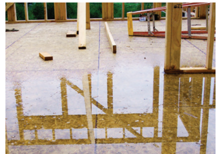
Jobsites in the Pacific Northwest are commonly exposed to extended wet conditions. Because pointSIX Flooring offsets the effects of moisture, Lincoln Creek Lumber customers are able to avoid the extra costs of sanding subfloor edges.
